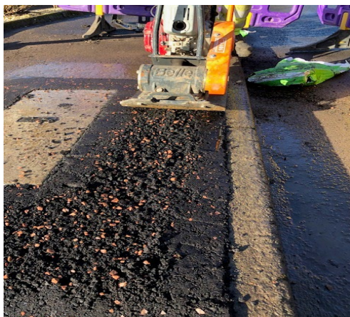
Decorative coloured chips can be added just prior to compaction if required
