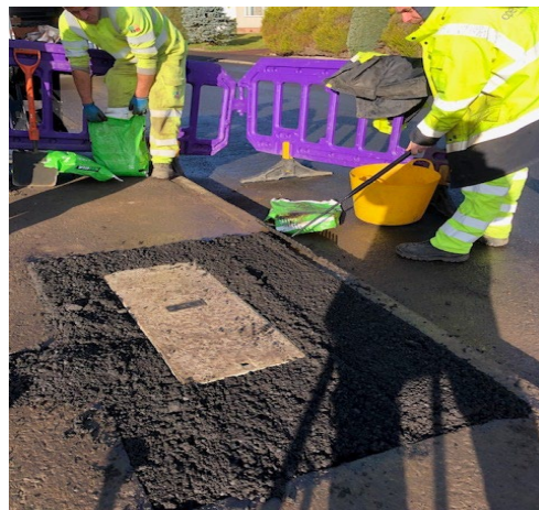
Viafix Quick HRA 15/10 AKA sand-carpet pre-compaction spreading
